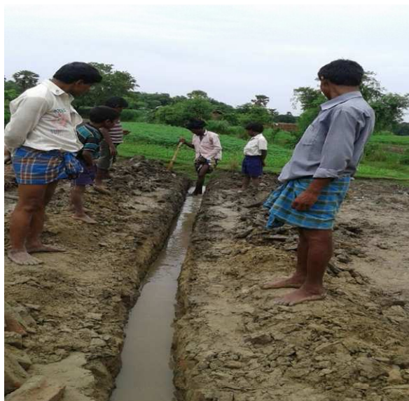
Drainage construction by the Community
